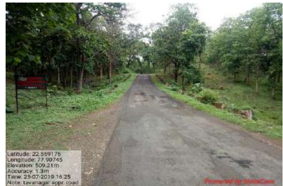
Figure 3-51 : Approach to Tawa Nagar
