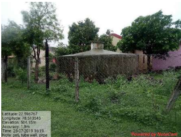
Figure 3-91 : Ground water Sump, Jhirpa
