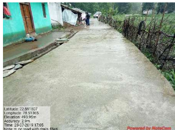
Figure 3-116 : Roads with one side drain, Fiferi
