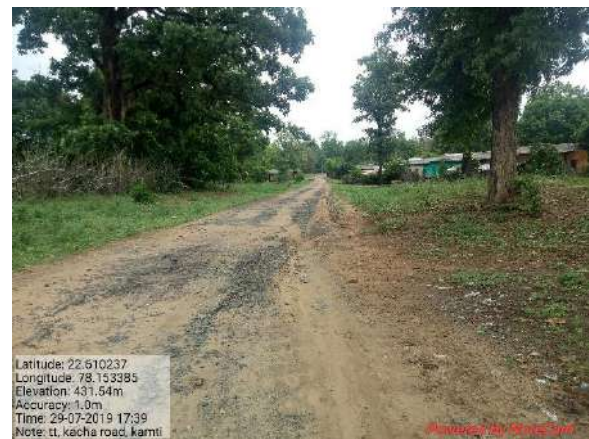
Figure 3-96 : Kacha Road, Kamti
