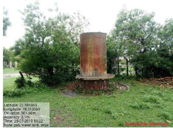
Figure 3-94 : Water Storage tank, Jhirpa
