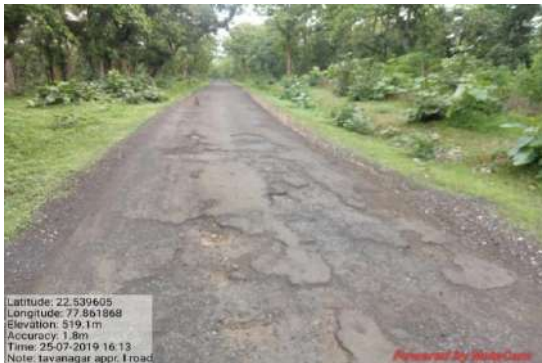
Figure 3-50 : Approach to Tawa Nagar
