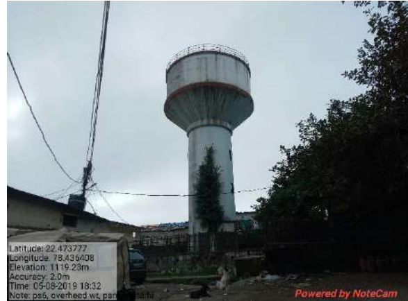
Figure 3-82 : Overhead Tank, Pachmarhi
