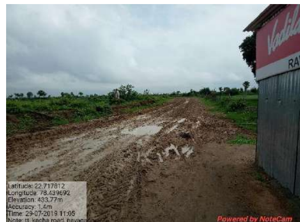
Figure 3-98 : Kacha Road, Nayagaon
