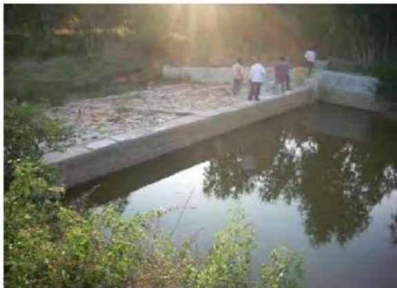
Figure 10. Check Dam Constructed at Malur Taluk
