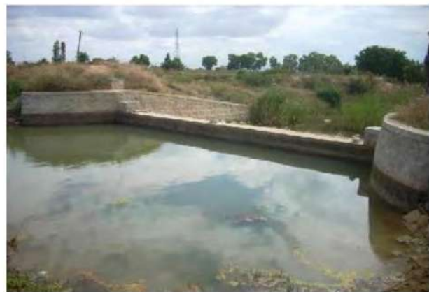
Figure 11. Percolation Tank Constructed at Malur Taluk
