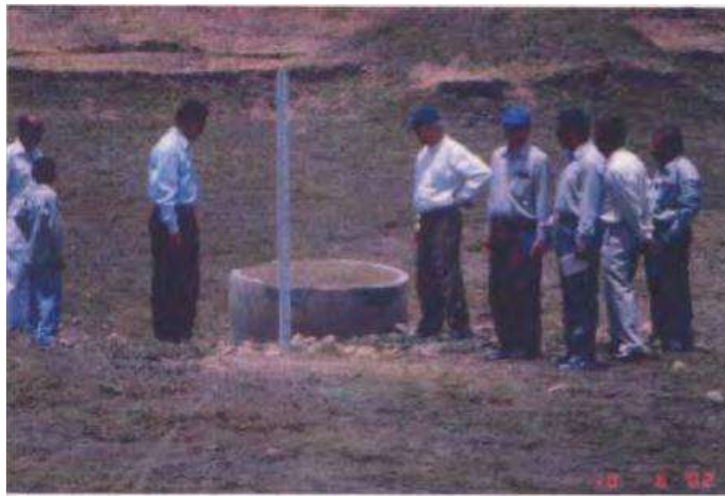
Figure 8. Recharge Shaft at Mendkichak District Dewas
