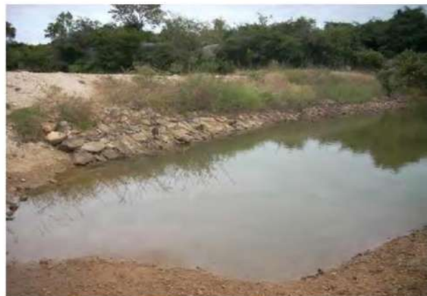
Figure 12. Nala Bund constructed in Malur Taluk
