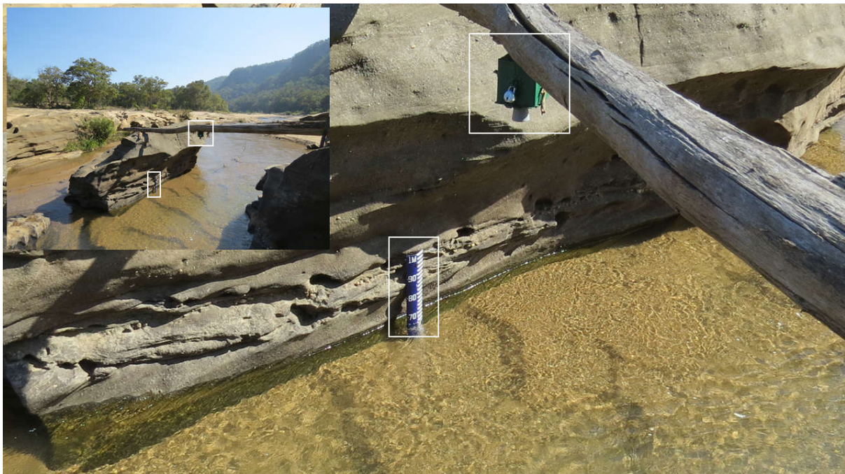
FIGURE 19 STAFF GAUGE AND WLR INSTALLATION AT DEHLIYA, DENWA RIVER
